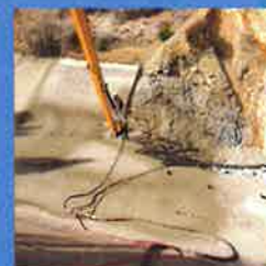
Shot crete work done at tunnel (AFTER)
